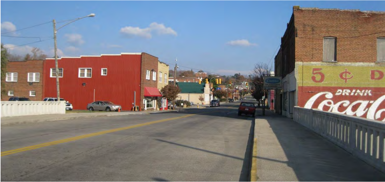
Washington Avenue & Jefferson Avenue Bridges: The bridges over Peak Creek are wide and lack buffers between traffic lanes and sidewalks.
